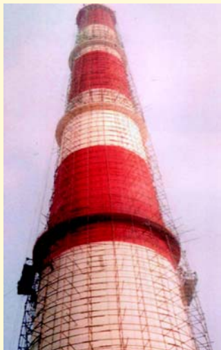
Fig. 10: A Chimney after repair & coating
