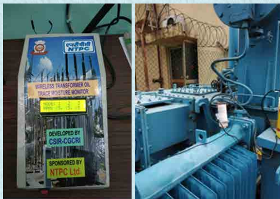
Moisture sensor receiver and transmitter system Installation work at NTPC, Faridabad plant
