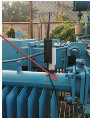
Sensor dip in transformer oil with data transmitter system
