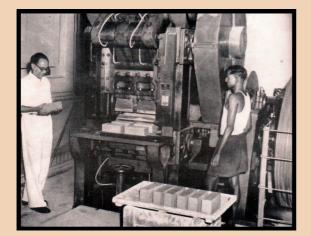
A 500-ton press for making refractory bricks in the Institute with 70-95% alumina contents.
